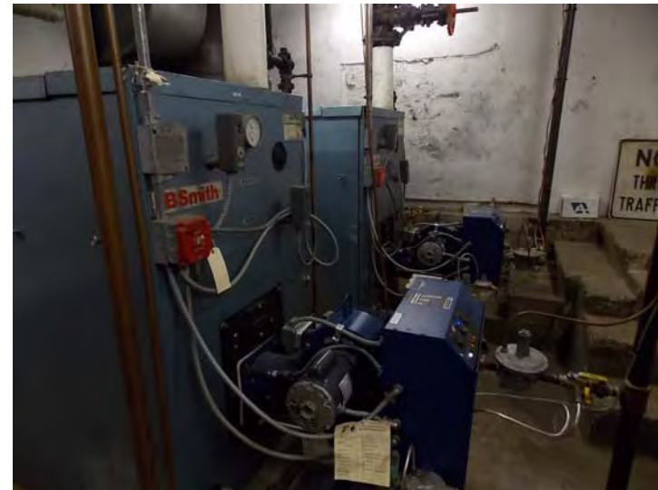
The central mechanical room includes a pair of dual fuel boilers used to produce hydronic heat and DHW.
