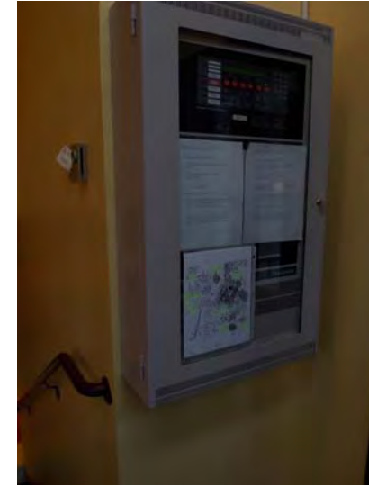
This is the fire alarm control panel (FACP).
