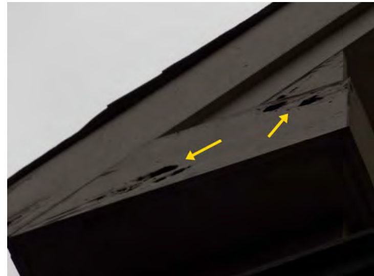
A close-up view of damaged wood trim.
