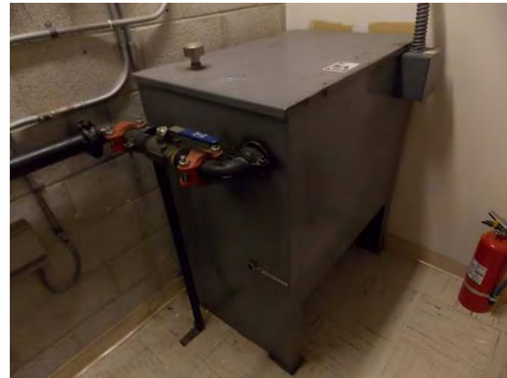
A view of the hydraulic elevator pump station.
