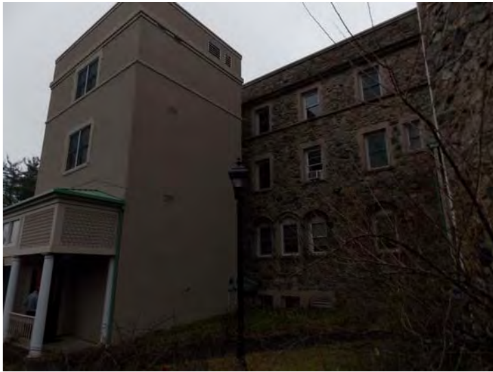
. The original building has stone exterior walls; the new wing is clad with synthetic stucco.
