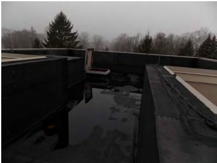
Ponding, which indicates inadequate drainage, was observed on sections of the membrane roof.
