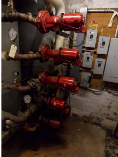
The hydronic circulating pumps.
