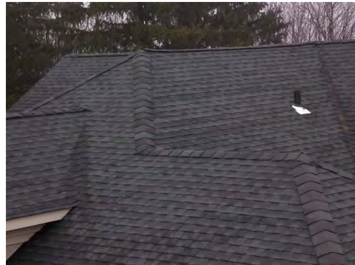
The newer wing roof is covered with asphalt shingles.
