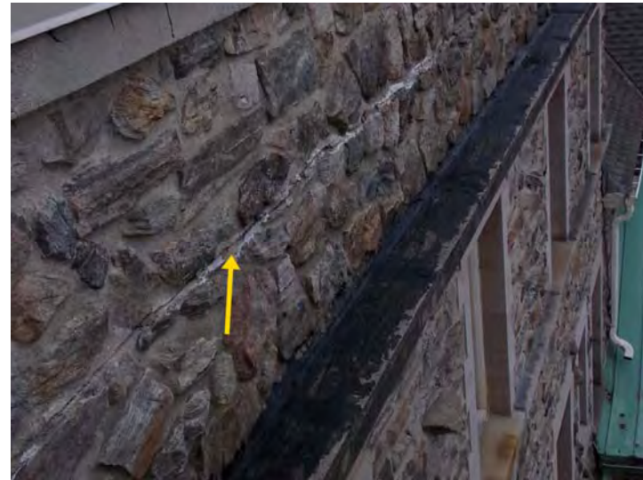
A score line (purpose unknown) exists in the stone exterior walls near the roof line.
