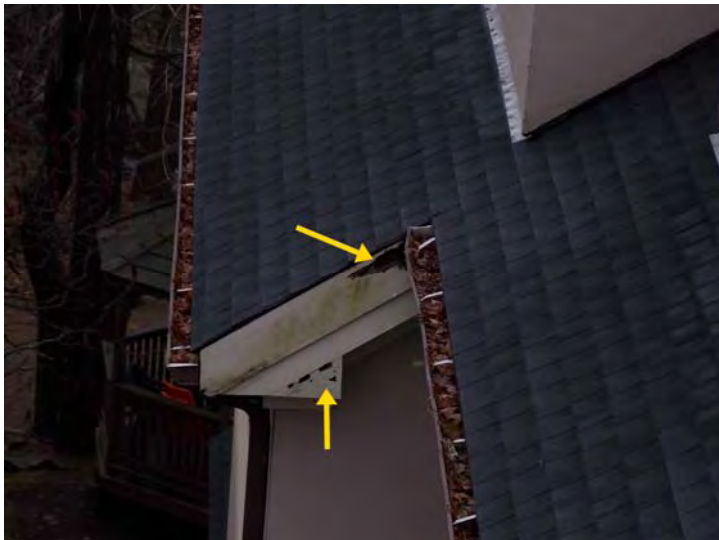
Sections of the wood trim have been damaged by insects and weather. Also, gutter guards are being considered to keep them clear of debris.
