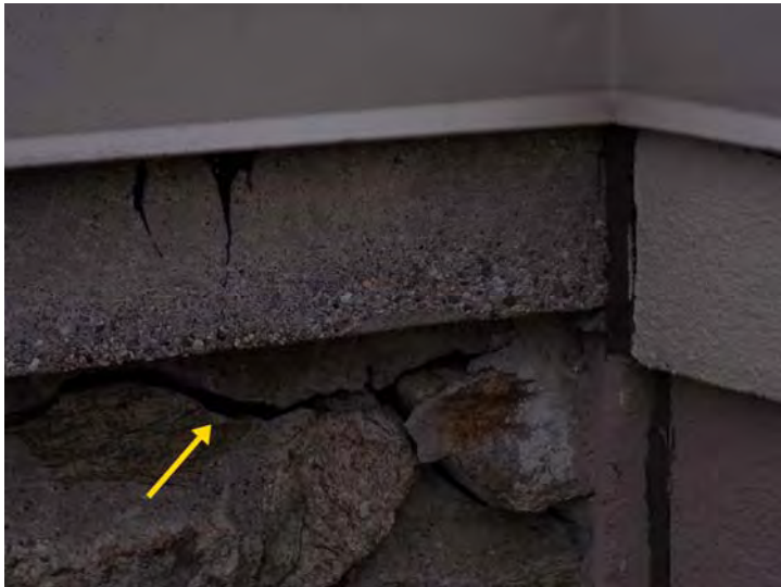
A close-up view of a section of missing mortar.
