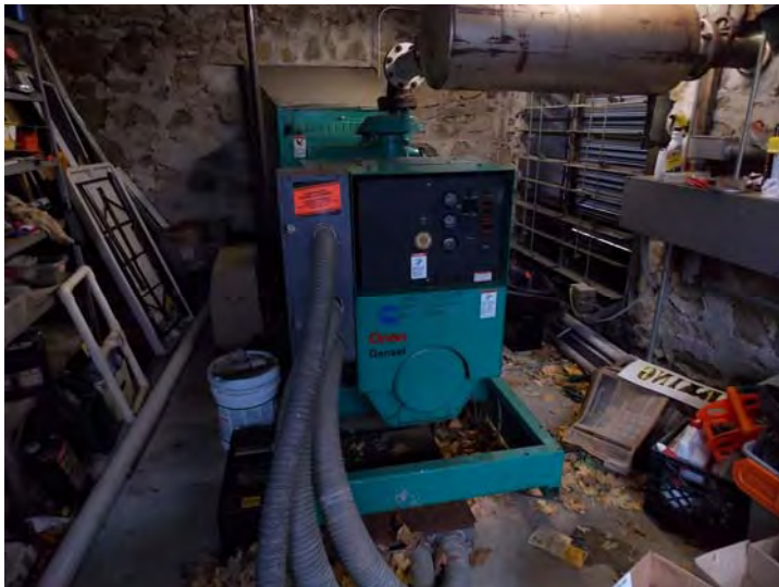
This diesel generator provides 125 kW of emergency power.
