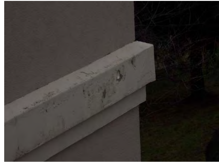
A close-up of a damaged section of synthetic stucco.
